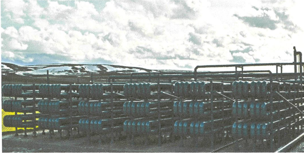
Figure 2: Biopipe Technology STP
